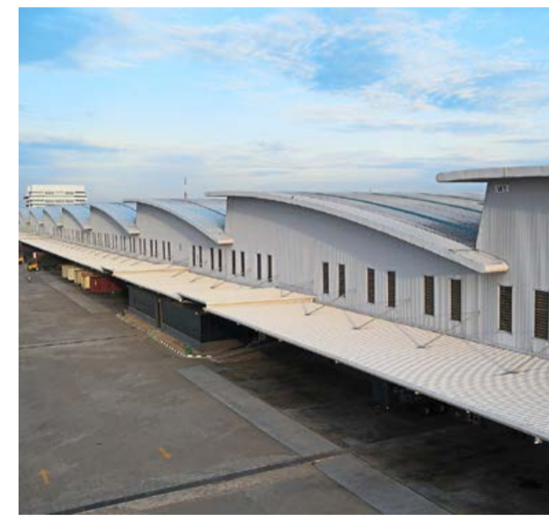
A side view of The 12 Waves illustrates the length and scale of the structure.
