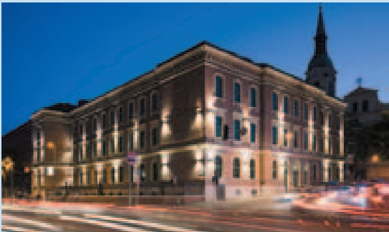
Bécsi Corner Office Building
