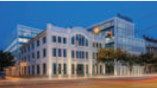
V47 - GTC White House Office Building, Budapest
