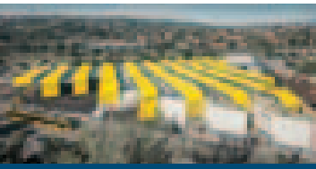
Budafok Tram Depot
