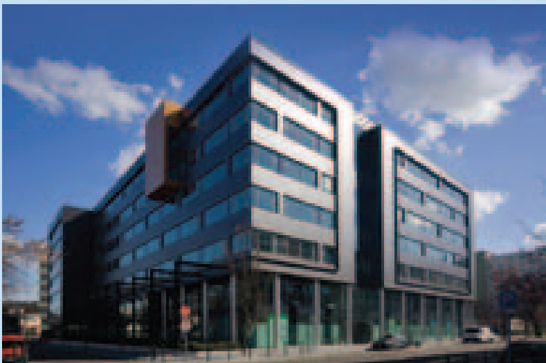
Green House Office Building, Budapest
