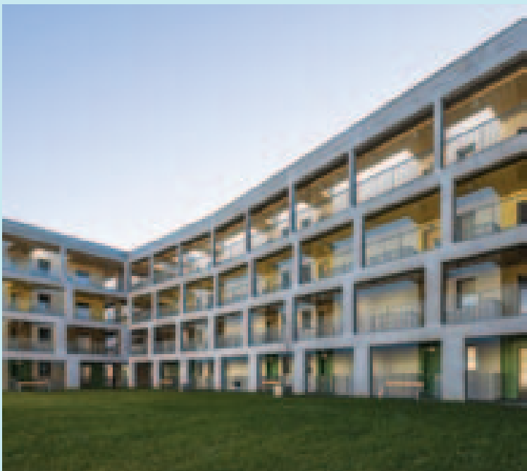
100 flats passive house, Budapest
